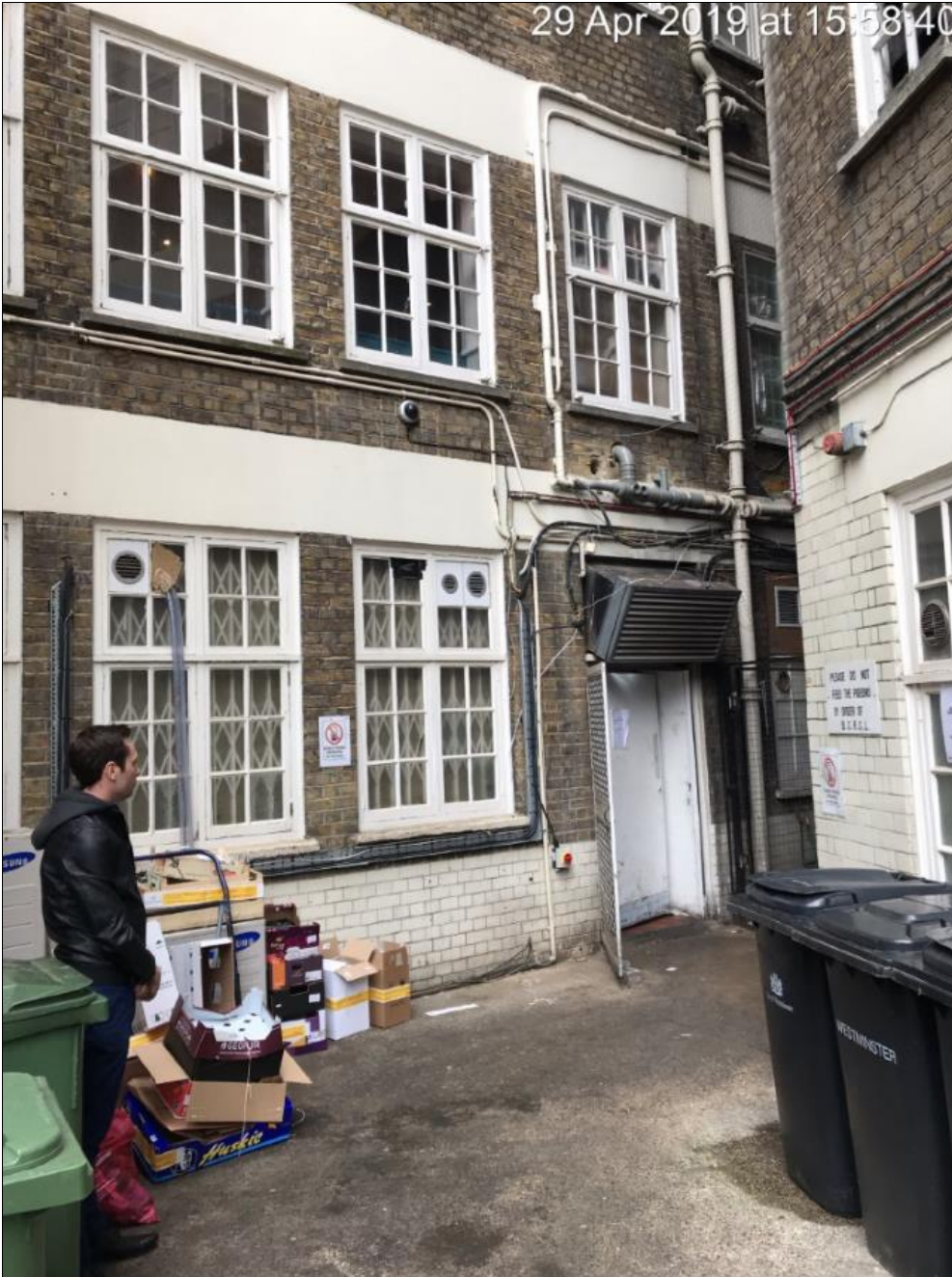
Cold room condenser removed – photograph taken 29 April 2019
